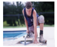
Floor & Wall Tiling
